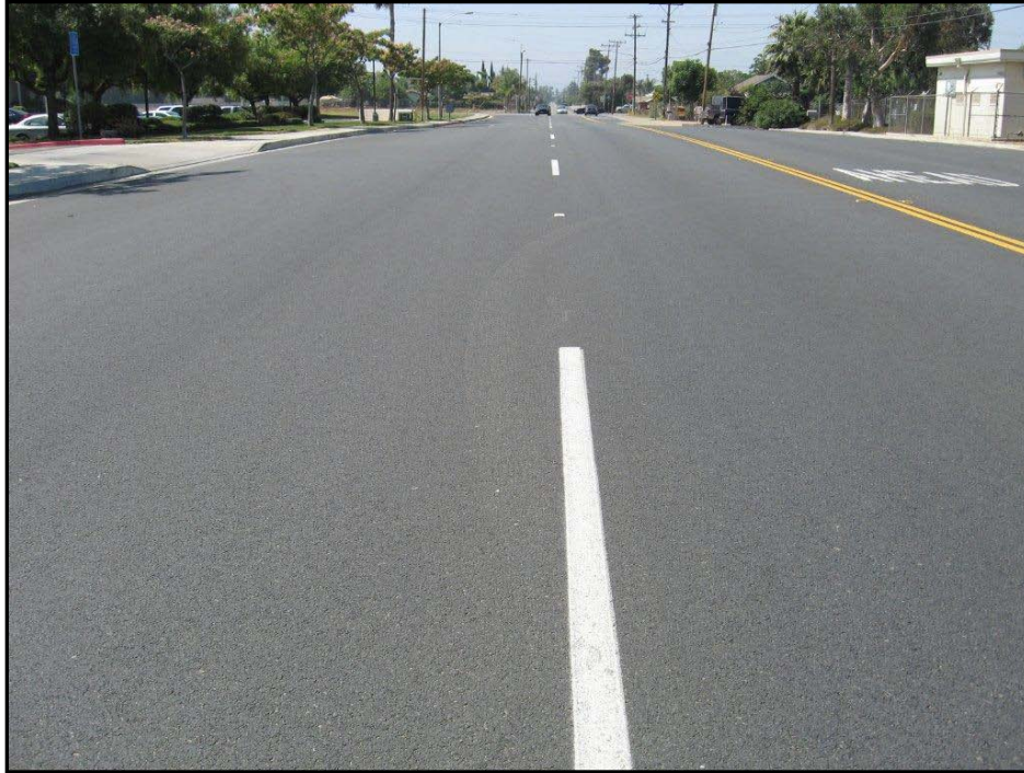
Figure 1A. PCI=98 (Excellent Condition)
