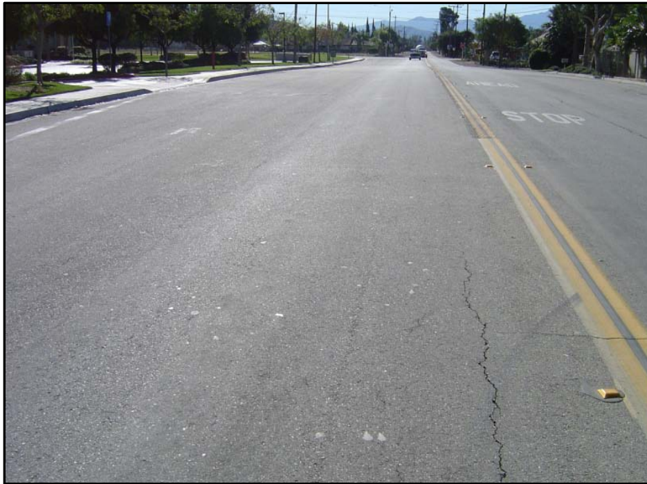
Figure 1C. PCI=78 (Good Condition)
