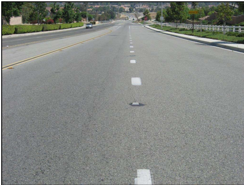
Figure 1B. PCI=85 (Very Good Condition)
