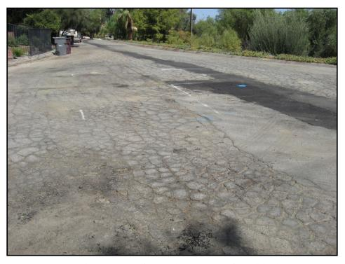
Figure 2F. PCI<10 (Very Poor Condition)
