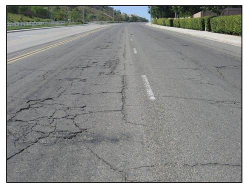
Figure 2E. PCI=30 (Poor Condition)
