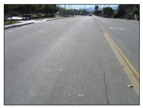
Figure 2C. PCI=78 (Good Condition)
