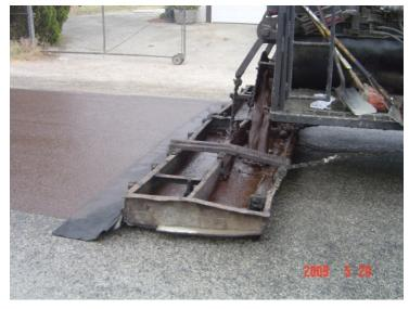
Figure 17. Spreading of slurry
