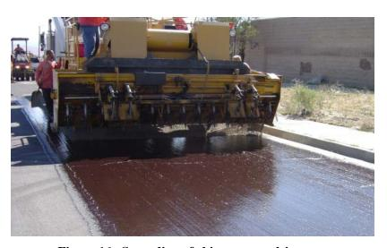
Figure 16. Spreading of chip over emulsion
