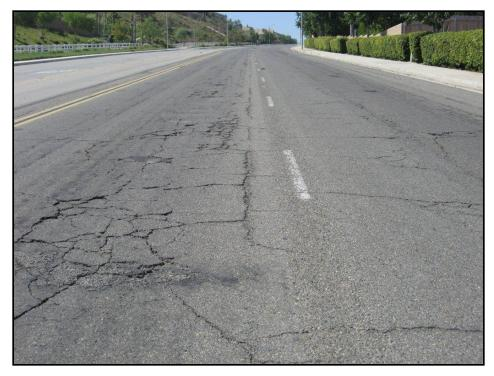
Figure 2E. PCI=30 (Poor Condition)
