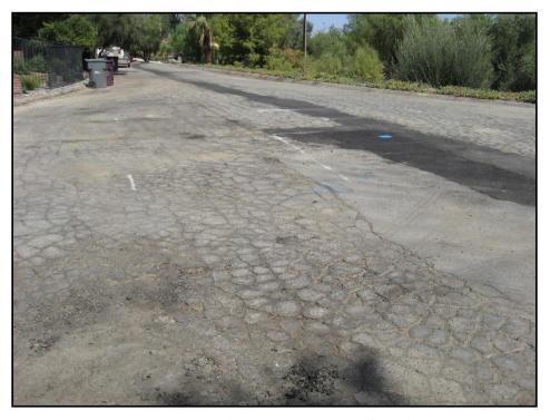
Figure 2F. PCI<10 (Very Poor Condition)
