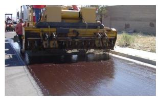
Figure 18. Spreading of chip over emulsion.
