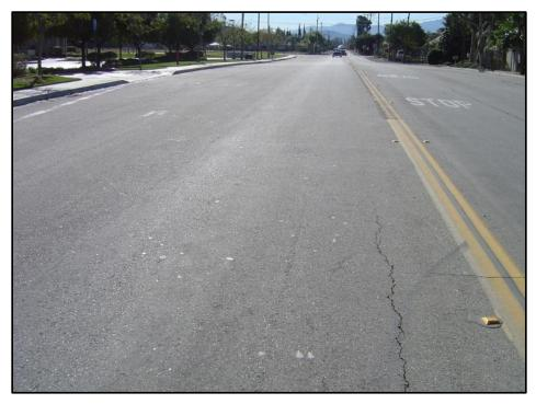
Figure 2C. PCI=78 (Good Condition)
