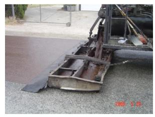
Figure 19. Spreading of slurry.
