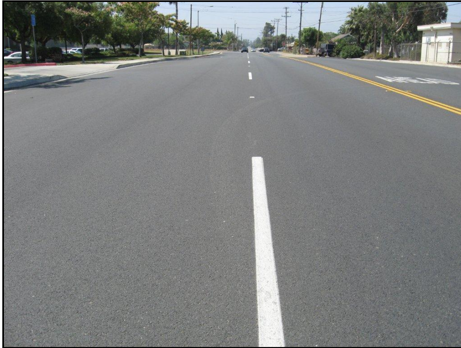
Figure 11A. PCI=98 (Excellent Condition)
