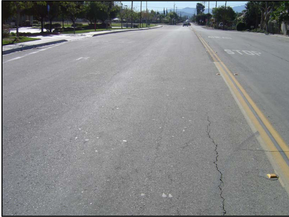
Figure 11C. PCI=78 (Good Condition)
