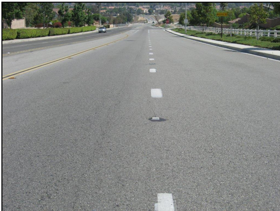
Figure 11B. PCI=85 (Very Good Condition)
