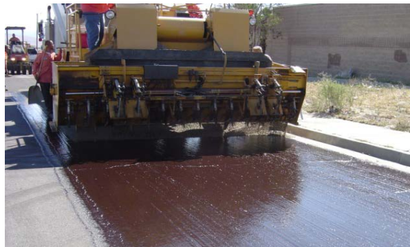
Figure 19. Spreading of chip over emulsion.
