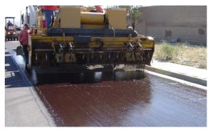
Figure 16. Spreading of chip over emulsion.
