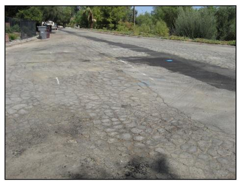
Figure 8F. PCI<10 (Very Poor Condition)
