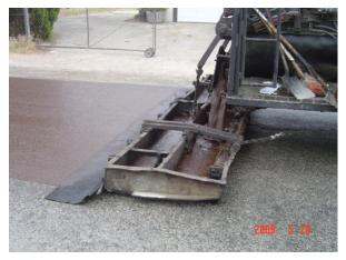
Figure 17. Spreading of slurry.
