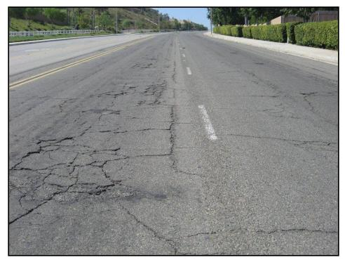
Figure 8E. PCI=30 (Poor Condition)
