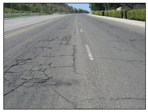
Figure 8E. PCI=30 (Poor Condition)
