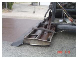
Figure 17. Spreading of slurry.
