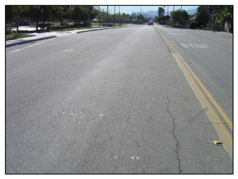
Figure 8C. PCI=78 (Good Condition)
