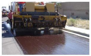
Figure 16. Spreading of chip over emulsion.
