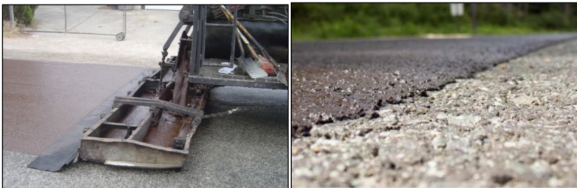
Figure 23. Spreading of Micro-surface Slurry
