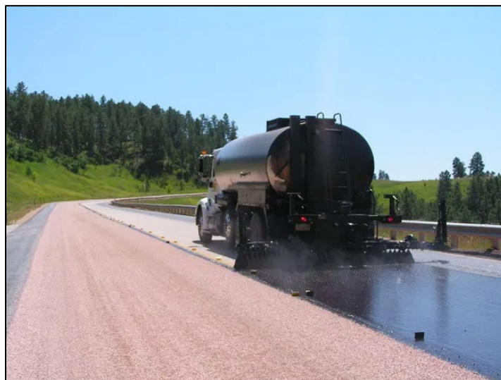
Figure 21. Chip Seal (slurry emulsion applied on right, chips applied on left)
