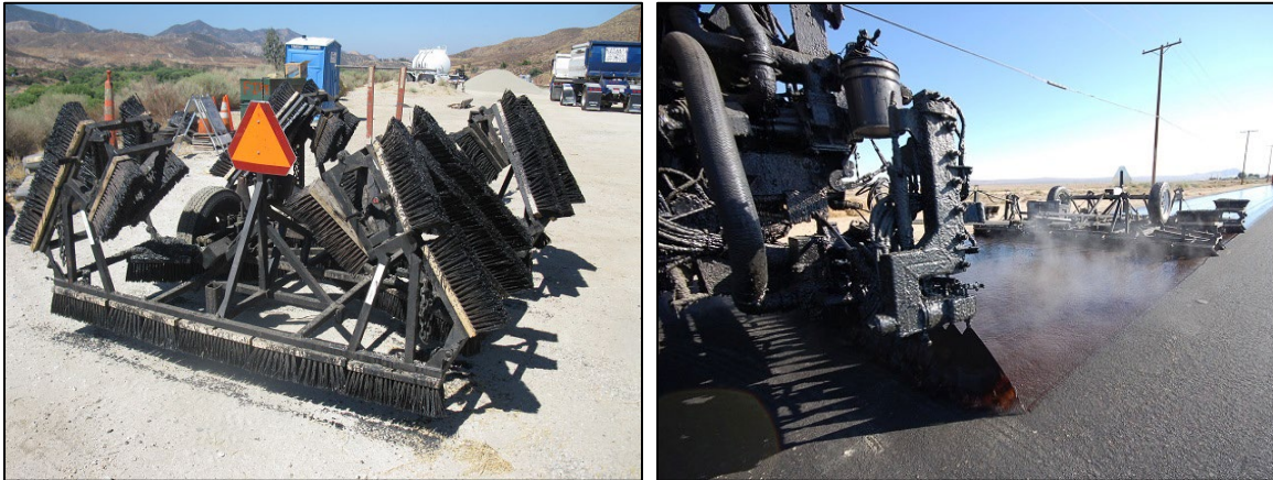
Figure 22. Scrub Seal (brooms on left, in use on right)
