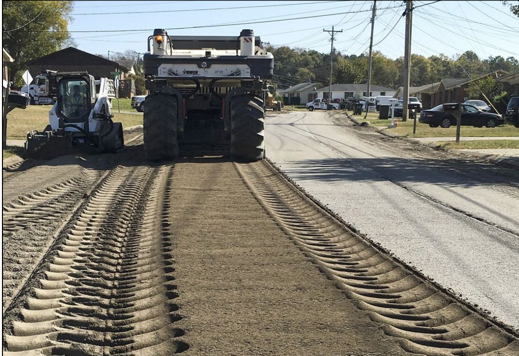
Figure 26. Full Depth Reclamation (FDR)
