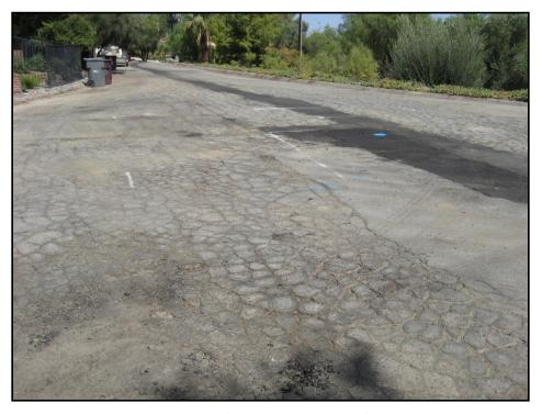
Figure 2F. PCI<10 (Very Poor Condition)
