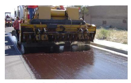
Figure 16. Spreading of chip over emulsion
