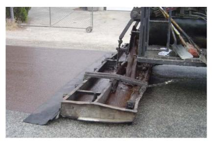
Figure 17. Spreading of slurry
