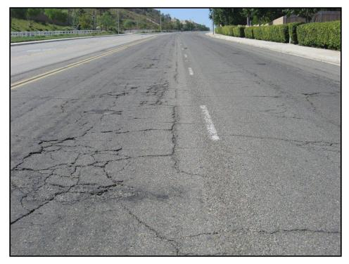
Figure 2E. PCI=30 (Poor Condition)
