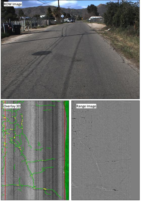
Figure 10F. PCI=38 (Poor Condition)
