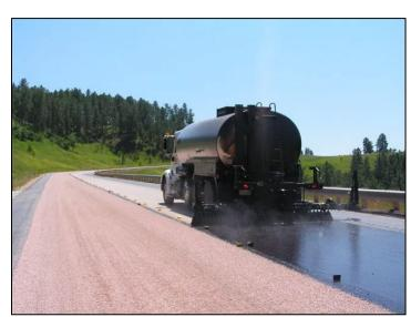
Figure 21. Chip Seal (slurry emulsion applied on right, chips applied on left)
