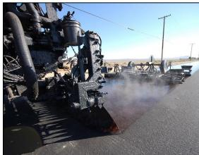
Figure 22. Scrub Seal (brooms on left, in use on right)
