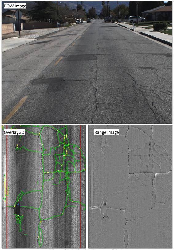
Figure 10G. PCI=26 (Poor Condition)
