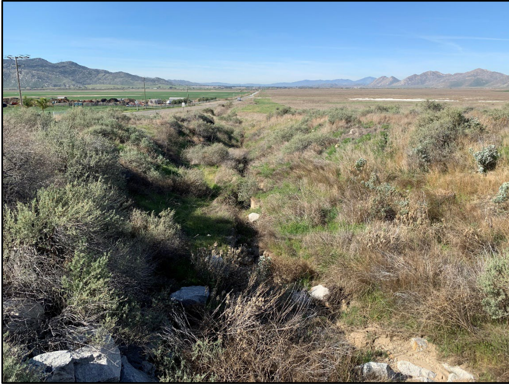
Figure 4-1 – Grasses and Brush in channel and overbank Downstream
