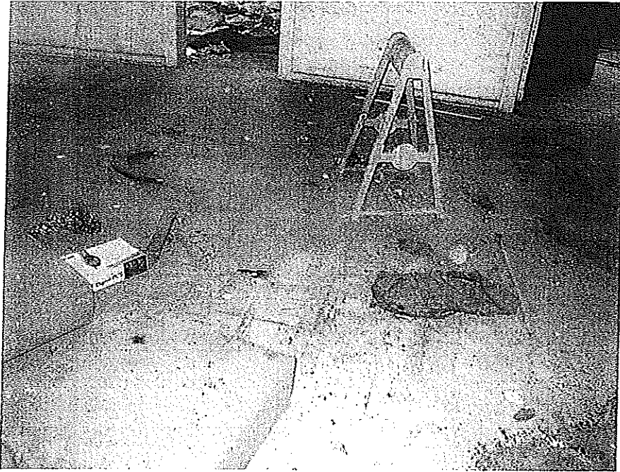
Photograph 1- illustrates the interior of the house living room, the ACM floor tile at 18050 Rice Road, Desert Center.
