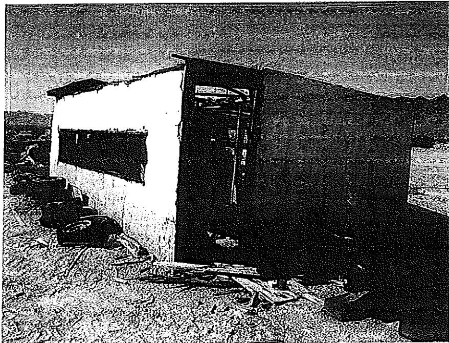
Photograph 4- illustrates exterior of agricultural building at 18050 Rice Road, Desert Center.
