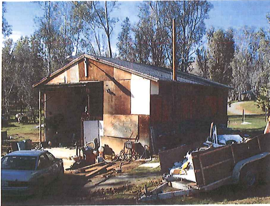
Photograph 1- illustrates the front exterior of the barn/workshop at 21665 Eucalyptus Lane, Perris.
